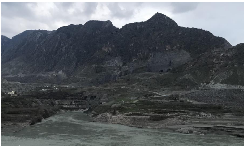
The unfinished Bekhme Dam. (2020)
