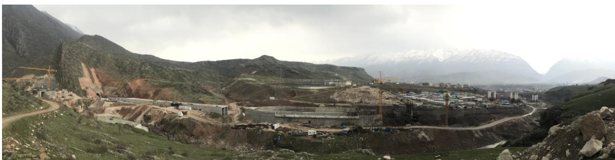
Construction site of Deraluk-Reshawa Dam. (2020)
