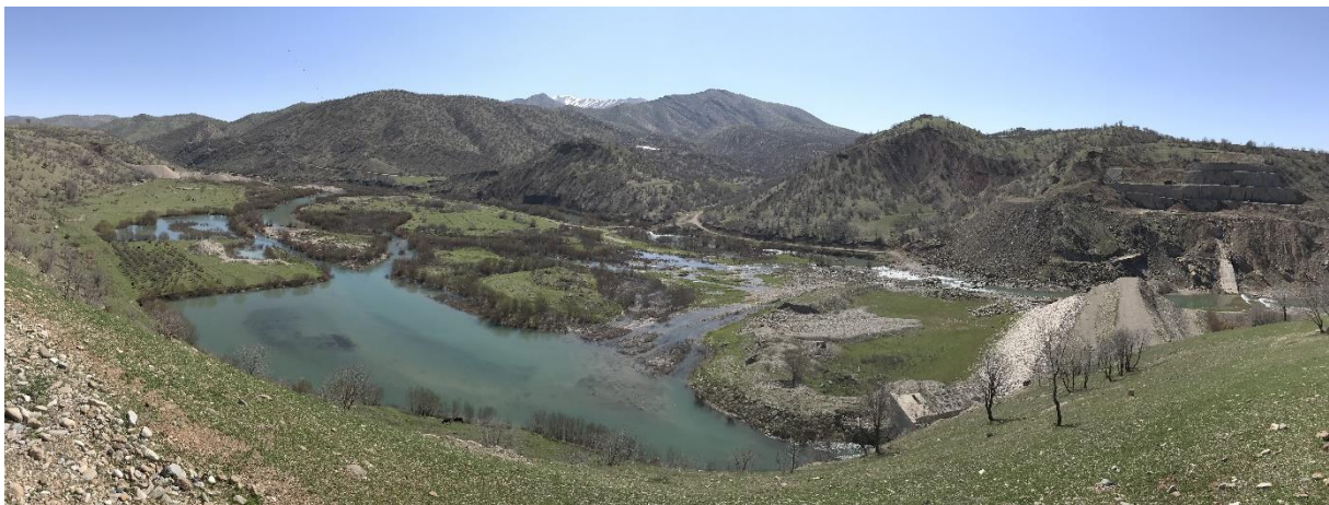
Destruction of the river as a consequence of gravel mining, behind the Zalan Dam in-construction (on the right side). (2020)
