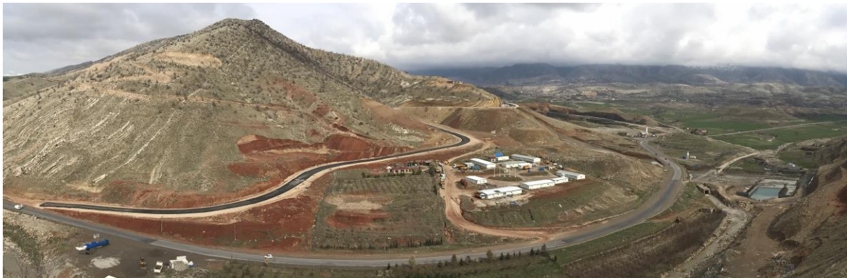
Construction site of Gomaspan Dam. (2020)
