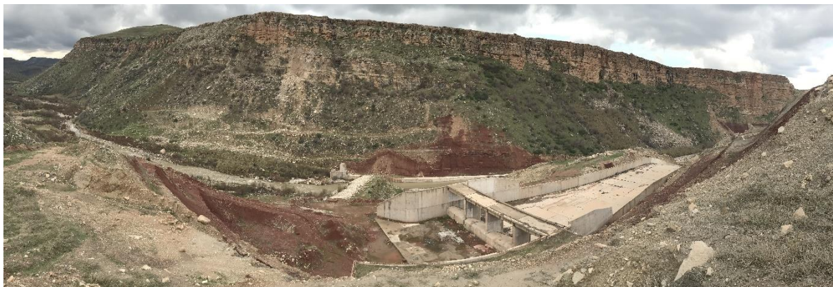
Construction site of Surqashan Dam. (2020)
