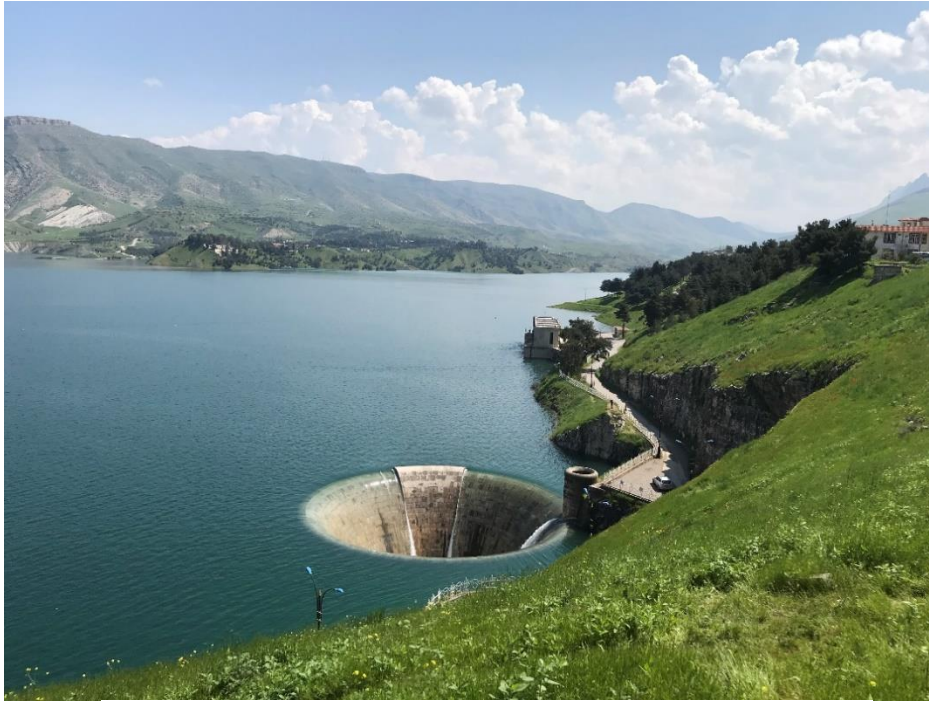
The spillway of the Dukan Dam in Iraq in April 2019, when the reservoir reached its highest level in 31 years. (2019)
