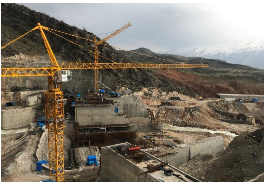
Deraluk Reshawa Dam under construction. (2020)
