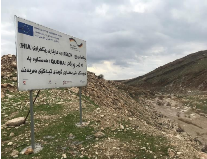
Sign at the new construction site of Basarah Dam. (2020)
