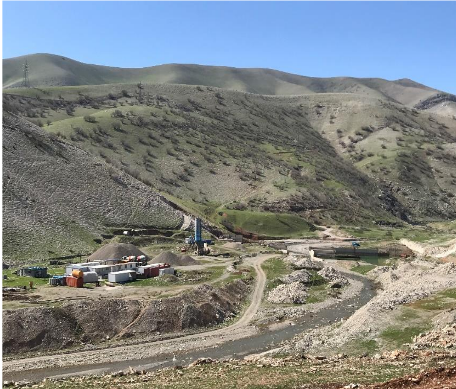
Construction site of Chaq Chaq 2 Dam. (2020)
