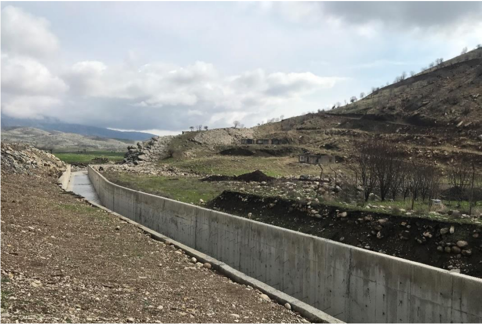
Canals of the Gomaspan Dam under construction. (2020)
