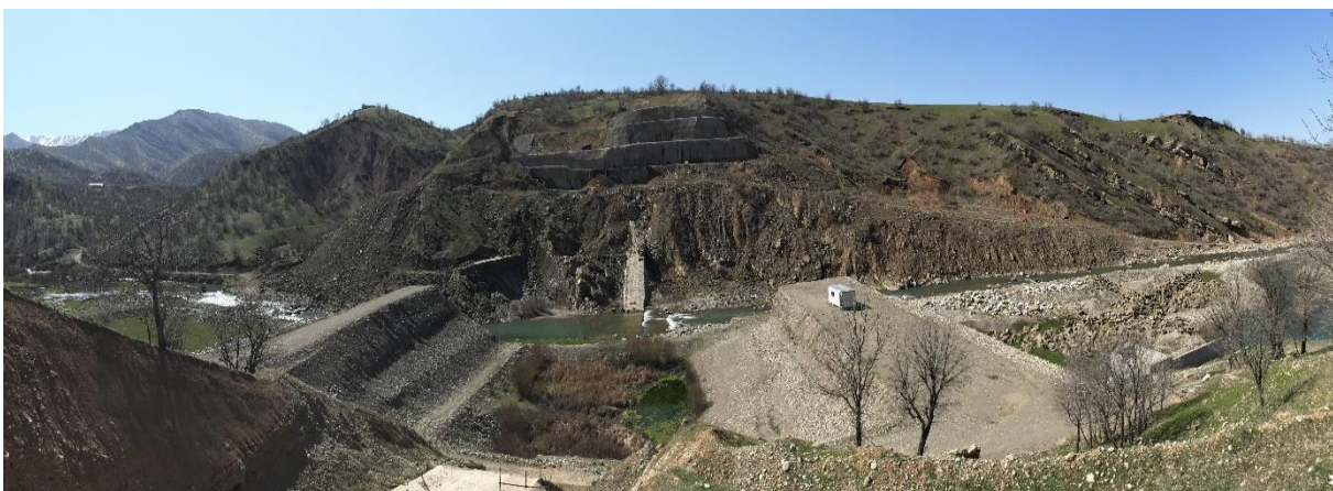
Construction site of Zalan Dam. (2020)
