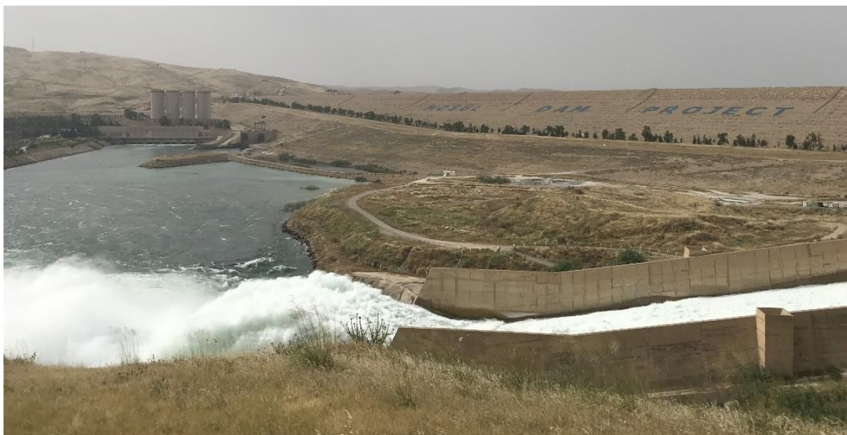
Mosul Dam, the largest dam in Iraq, provides electricity to the city of Mosul. (2019)
